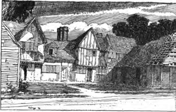
Cottages at Titmore Green, recently demolished.
